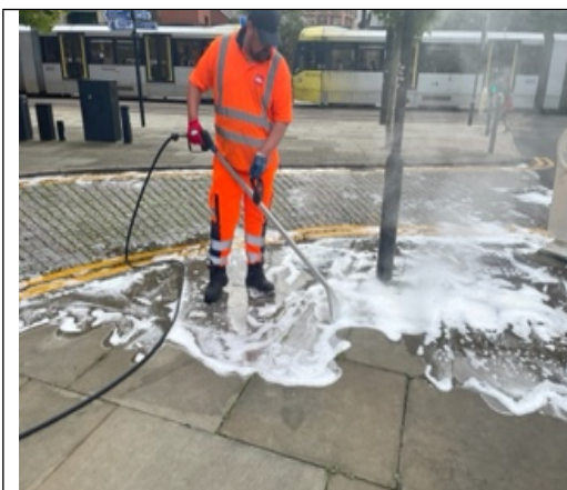
Operative applying hot foam treatment via lance
