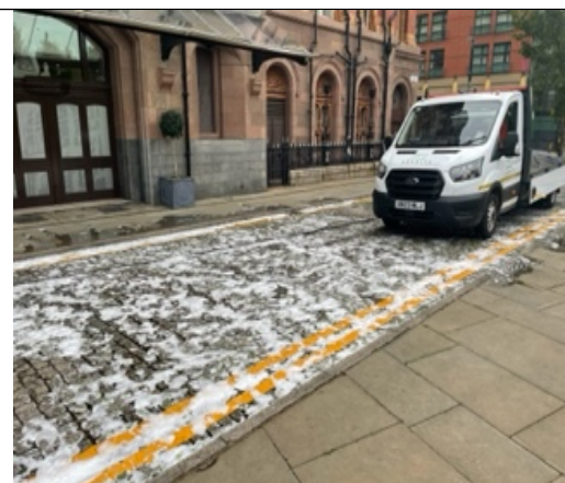
Van required to hold and transport the hot foam technology
